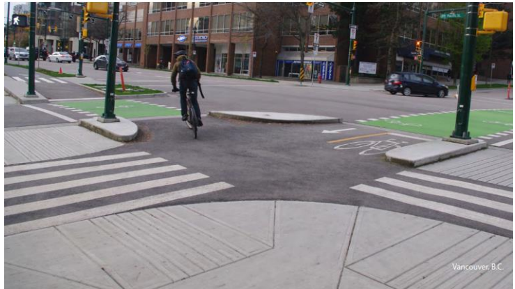
Protected intersection separates vehicles, cyclists, and pedestrians with physical barriers in Vancouver, BC. Image Retrieved from the BC AT Design Guide (2019).
