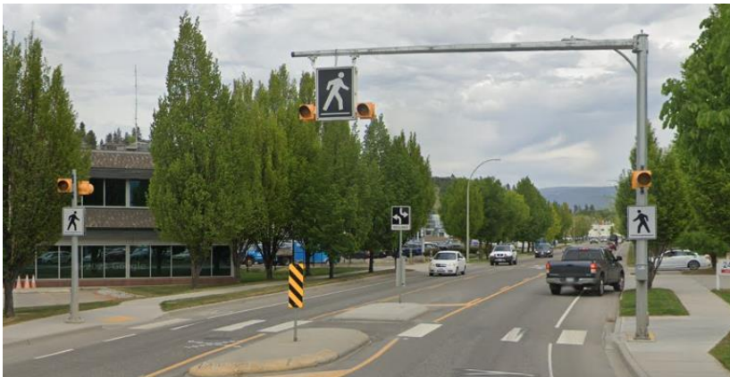
Pedestrian refuge example in Kelowna that includes overhead flashers. Source: Google Streetview.
