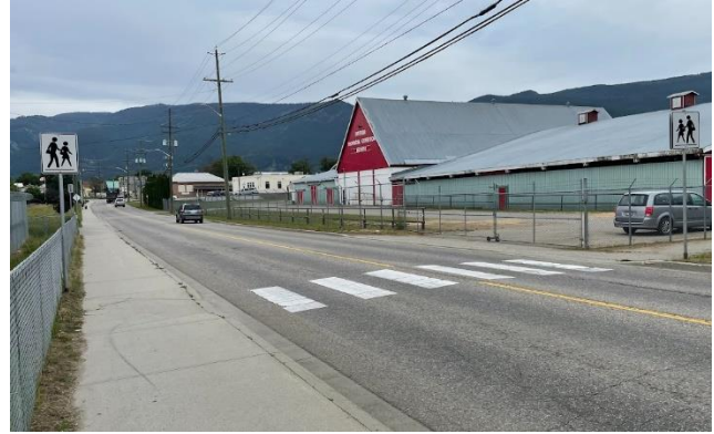
Wood Avenue is a candidate for a complete street cross-section that integrates a multi-use path.
