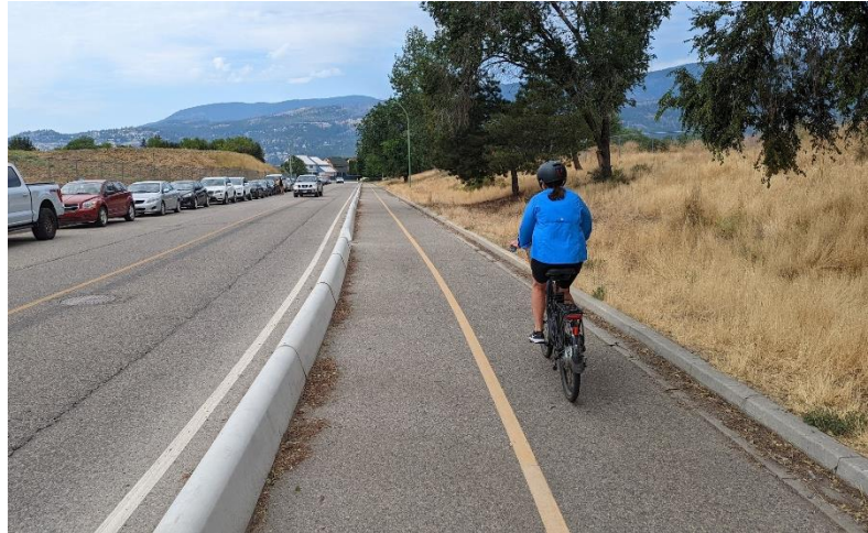
Example of a quick-build MUP in Kelowna, BC using line painting and pre-cast concrete barriers.
